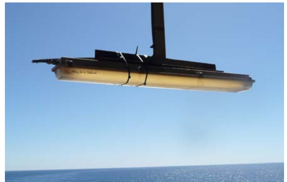
Examples of photos taken during NOPSA inspections. Corroded junction box on pump motor (left). Poorly maintained light fitting in process area (right).
