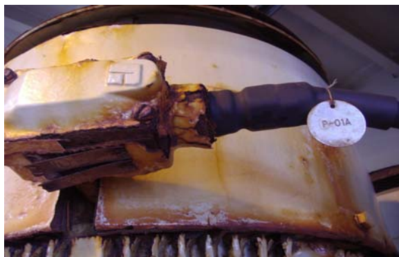
Examples of photos taken during NOPSA inspections. Corroded junction box on pump motor (left). Poorly maintained light fitting in process area (right).
