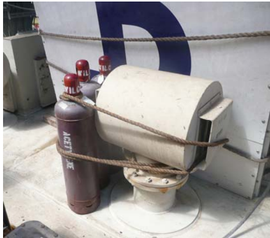
Acetylene bottles secured with rope – this is a dangerous way to store containers of flammable pressurised gases.
